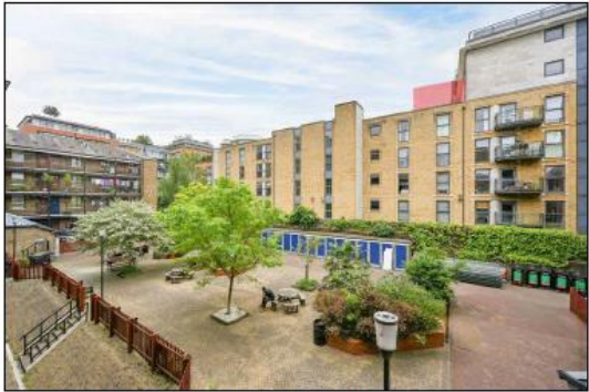
Above: View of Gatliff Close Communal Garden with zone of proposed extension in red
